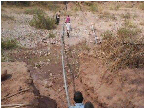
The original PVC pipes that make up the Mapongola pipeline in Nyaminyami are being replaced with stronger galvanised pipes ahead of the rainy season
